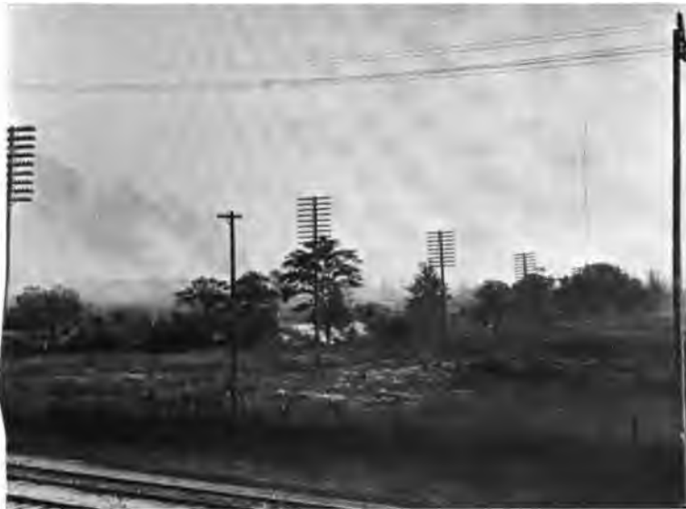
Fig. 1. Use of Messenger-Cable for High-Tension Crossing.*
